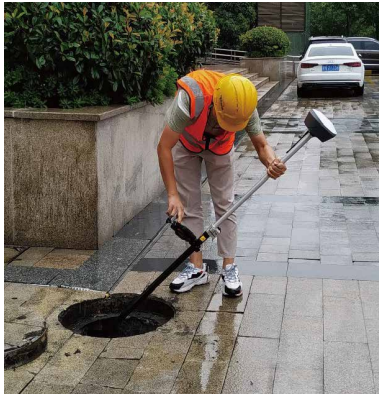
Figure 5.5 Tilt survey for a manhole
